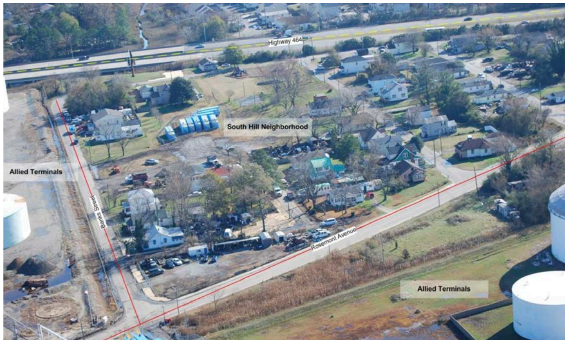
The Allied Terminals tank failure flooded the adjacent South Hill neighborhood and roadways with liquid fertilizer.
