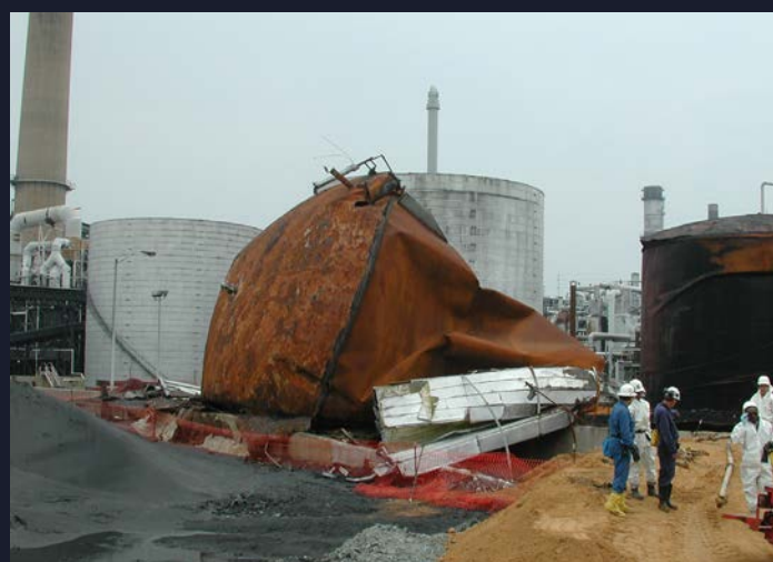
Collapsed tank from the Motiva Enterprises explosion.
